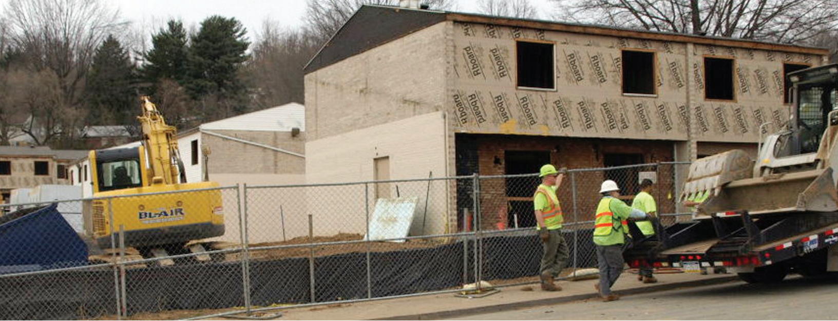
Above: Construction crews are moving quickly on the rehabilitation and renovation of 60 Cumberland Gardens apartments.
